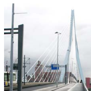
Erasmusbridge, Rotterdam multimodal bridge
