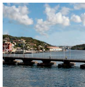
Ferrybridge, Willemstad: examp. movable bridge
