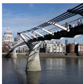
Millenium bridge London (lower freeboard 10,8m)
